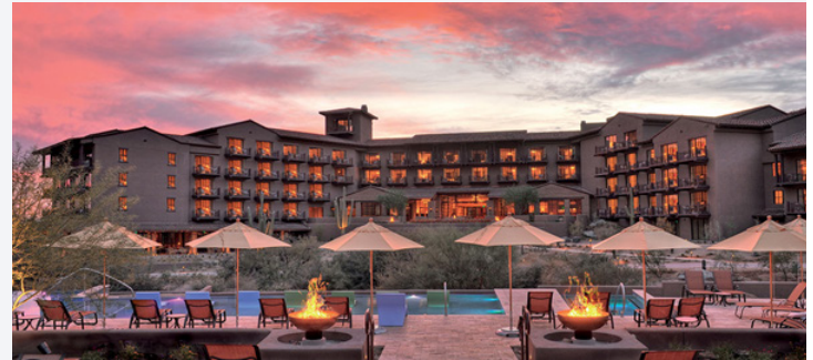
Provided ground-up HVAC and plumbing design services for this luxury 5-star resort framed against the Tortolita Mountains.
